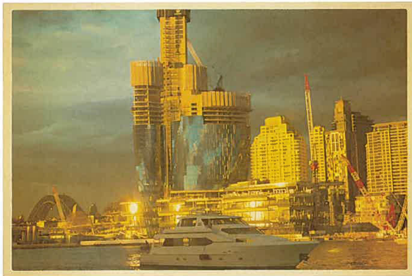
Crown's Barangaroo casino, under construction. RYAN STUART
